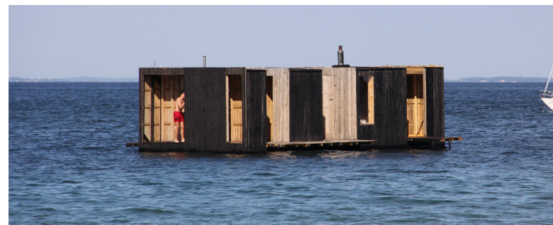
Flydende badepavillon 'PYR', RINTALA / EGGERTSSON ARCHITECTS
